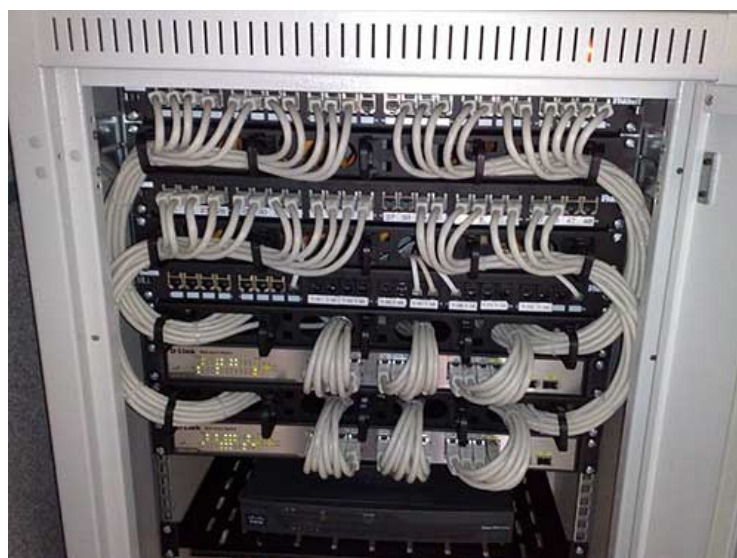
Figure 28 Rackmount Ethernet switches and patch panels may build several VLANs A couple of managed D-Link Gigabit Ethernet rackmount switches.... by Dsimic (Own work) from Wikipedia CC BY-SA 4.0
